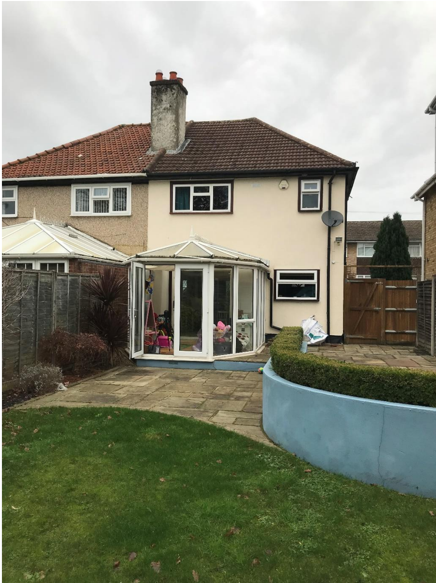
Rear elevation of No 67 with No 69 showing
