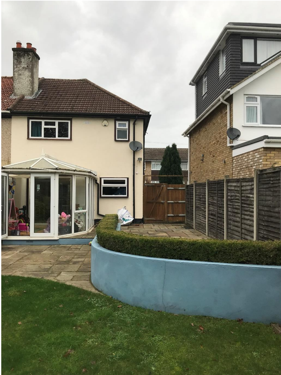
Rear elevation of No 67 with No 65 showing
