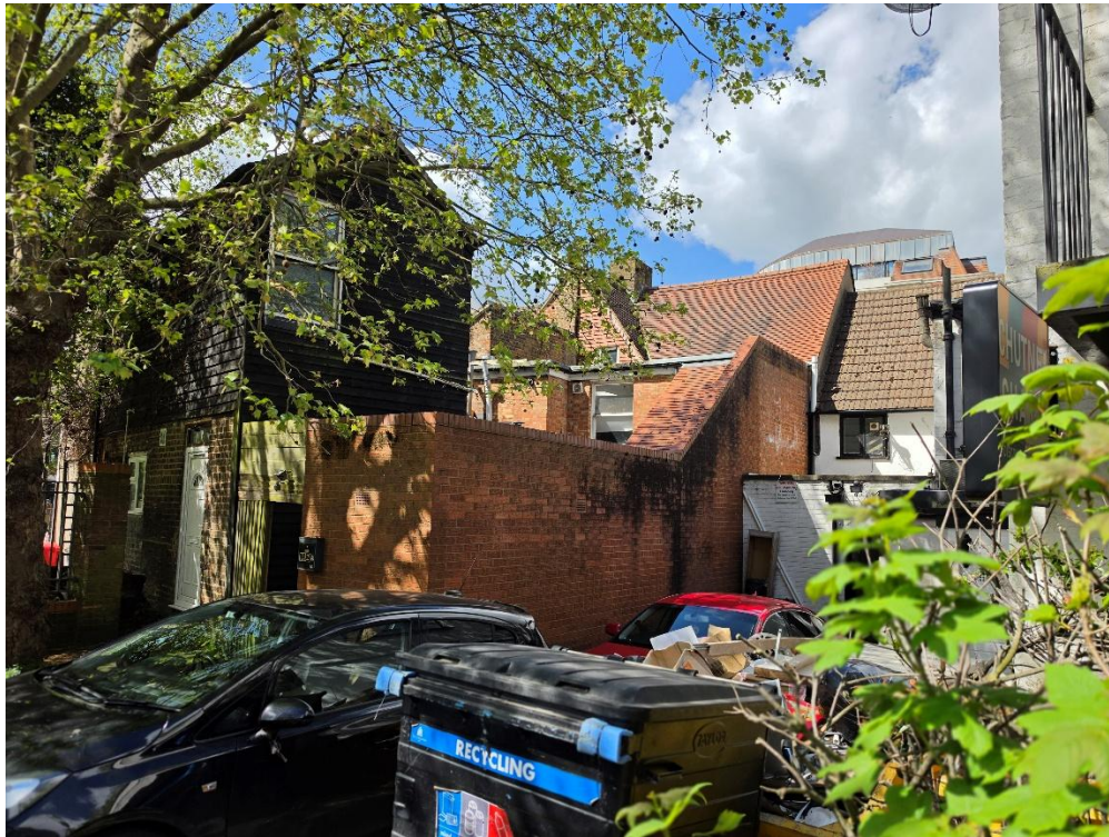
Figure-02 Rear View of the Site and its Surrounding
