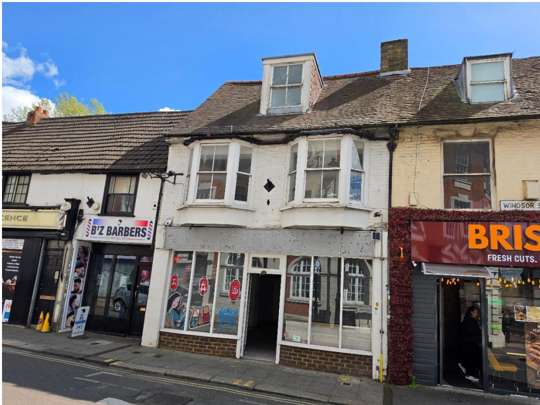
Figure-01 Front View of the Site and its Surrounding
