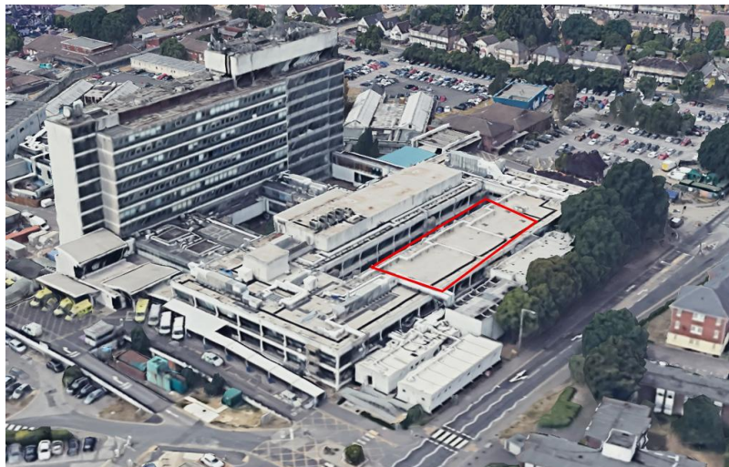
Figure 2 – Roof of proposed relocated SDEC where the proposed Air Handling Unit will be located (indicated in red)
