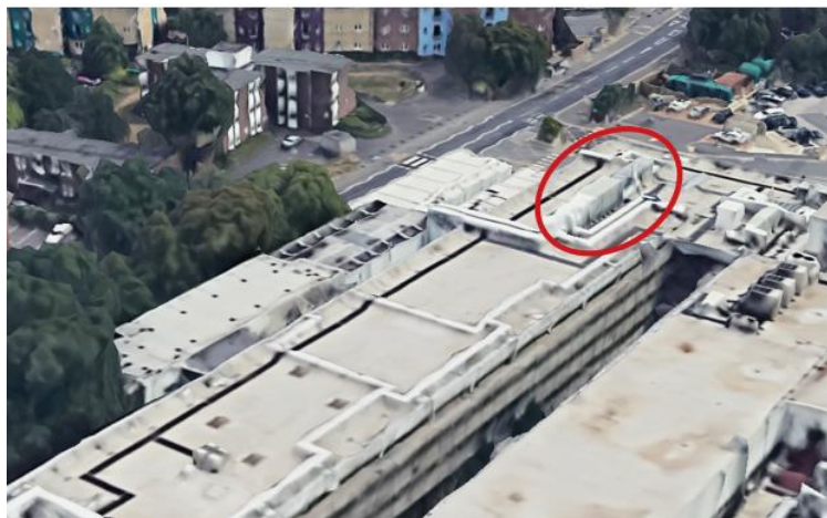
Figure 14 – The proposed AHU will be a similar height to the existing plant located further east on the Podium Building
