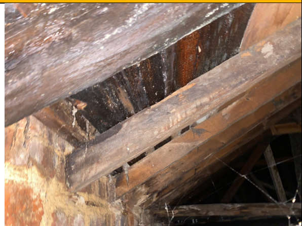
28 – Above 40.0/11.5 Leak from Slate Roof 01
