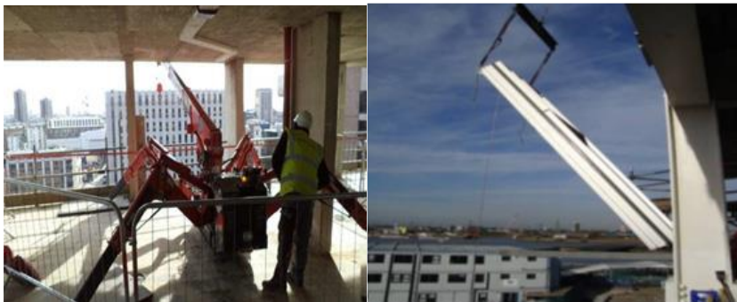
Figure 3-5: Example of spider crane from the floor above lifting panel into place
