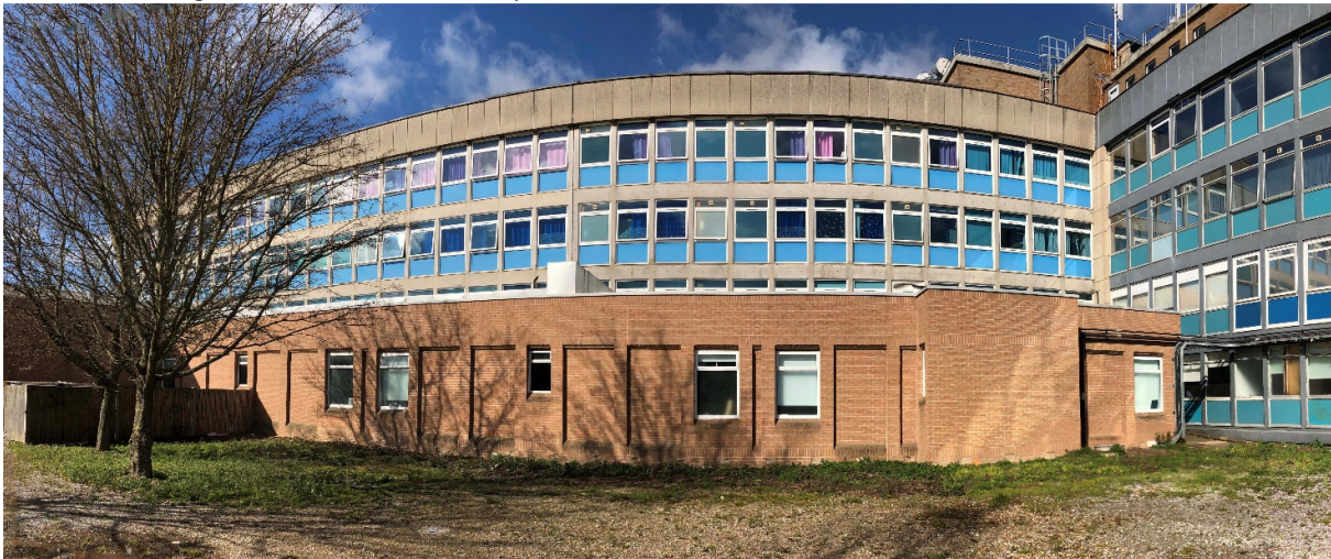
Panorama looking West across the site towards the maternity block where the new link connection will be formed
