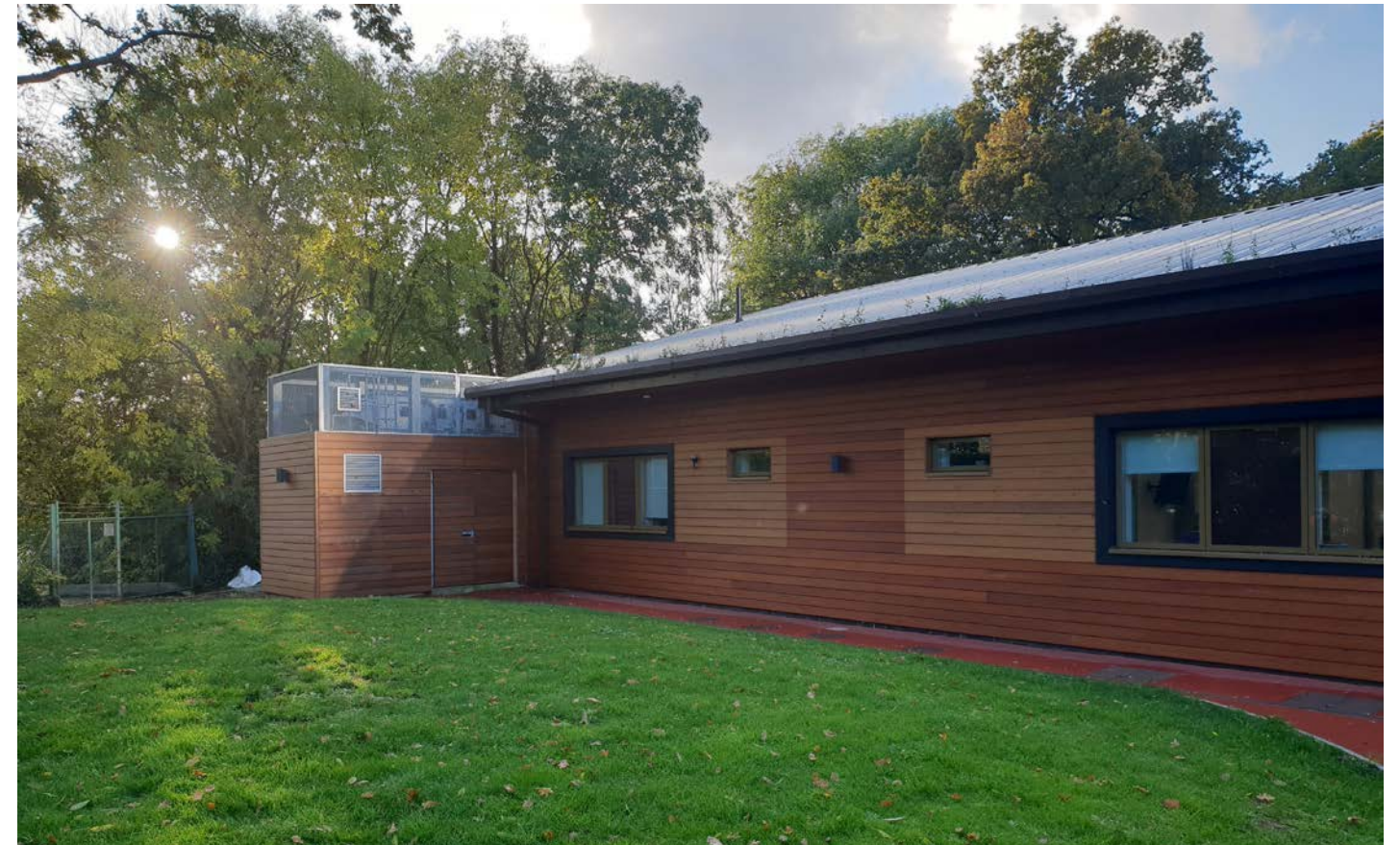
VIEW OF "THE POD" FROM THE EAST
