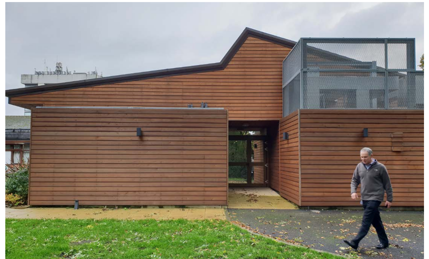
VIEW OF "THE POD" FROM THE SOUTH
