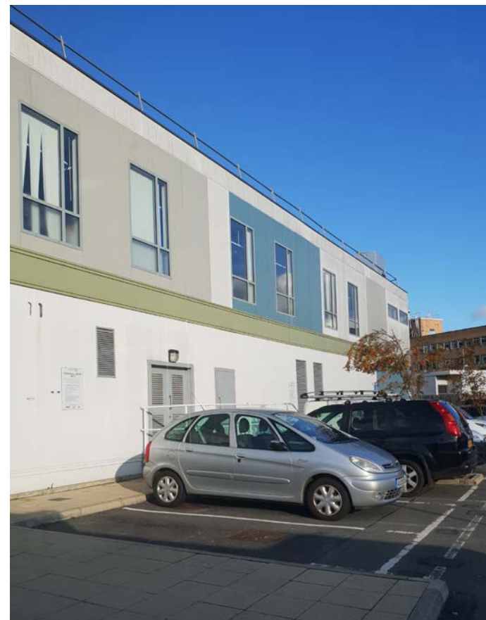
VIEW OF THE NIGHTINGALE AMU BUILDING
