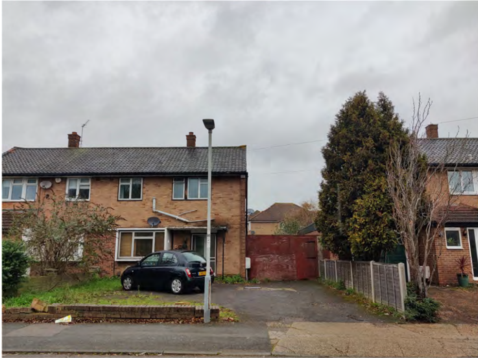
1. EXISTING SITE PHOTOGRAPH (FRONT ELEVATION)
