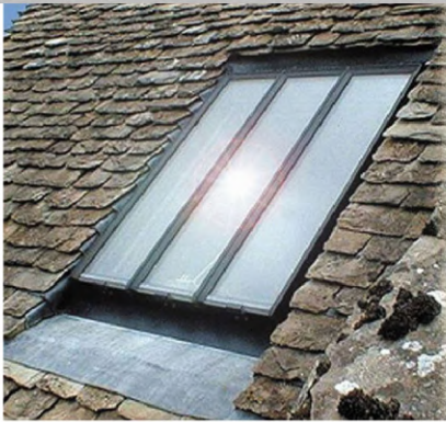
ROOF LIGHTS Conservation style rooflight "the rooflight company" or similar. To be flush with roofline. Both rooflights to be conservation style
