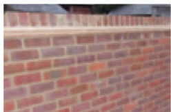
PHOTO SHOWING BRICK-ON-EDGE ON TILE CREASING Rear GF extension with concealed gutter
