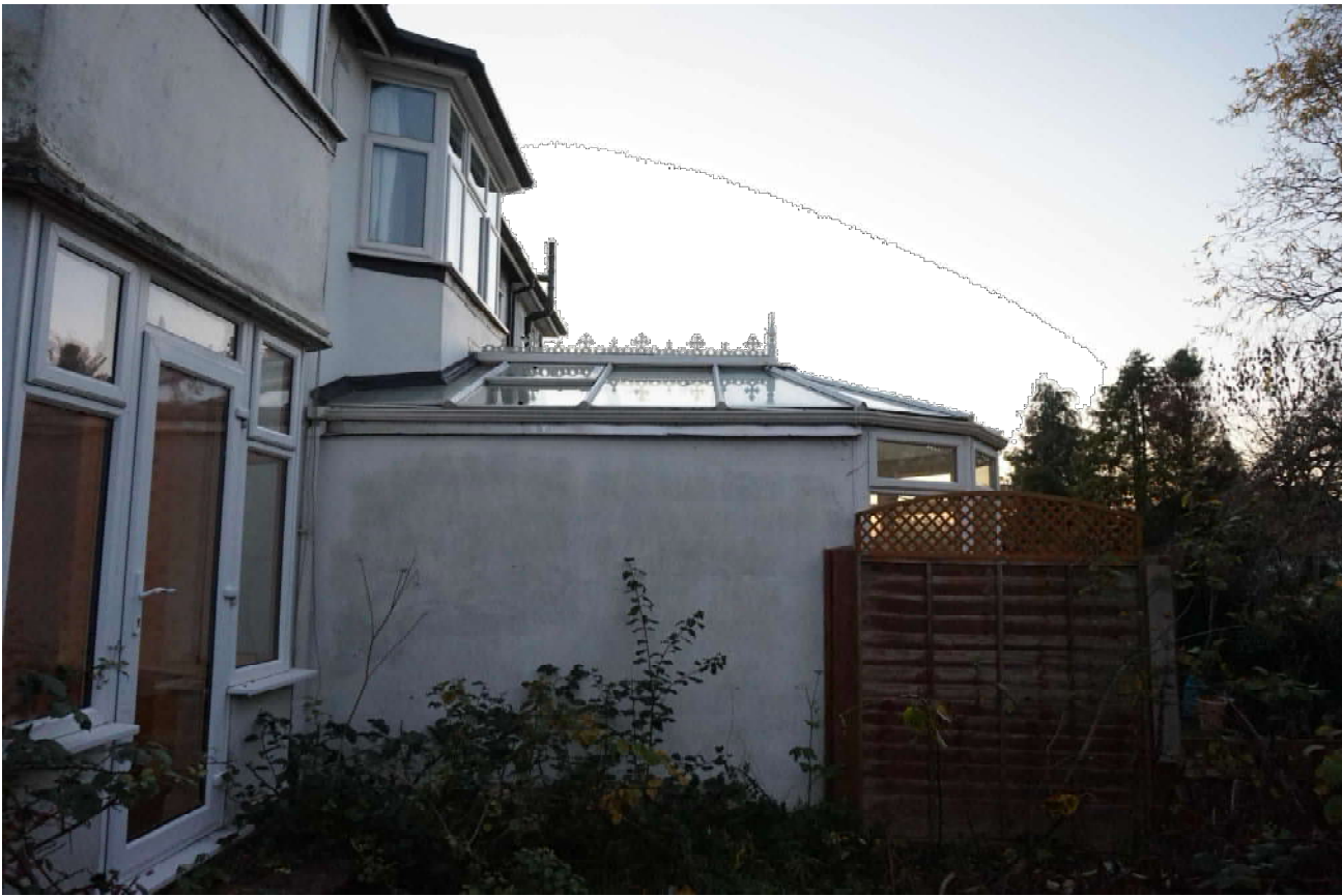
REAR VIEW SHOWING 35 BURWOOD CONSERVATORY FROM PATIO OF APPLICATION SITE.
