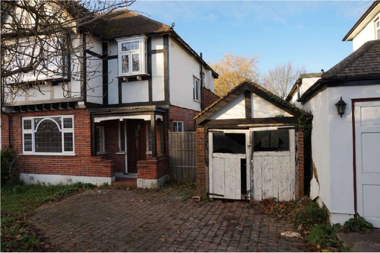
FRONT VIEW SHOWING GARAGE WHICH IS RUN DOWN AND IN VERY BAD CONDITON AND SIDE OF APPLICATION SITE
