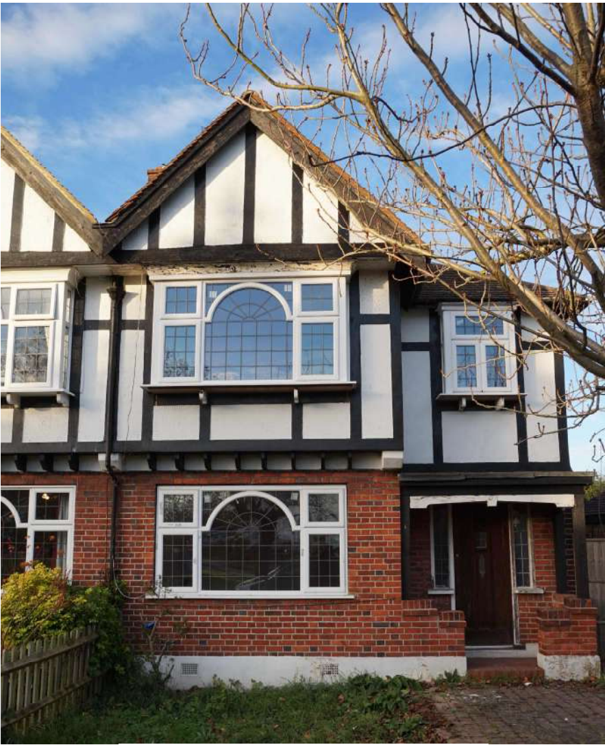
FRONT VIEW OF APPLICATION SITE
