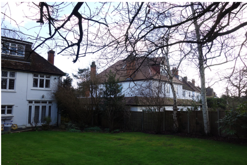
View from rear garden toward No.21
