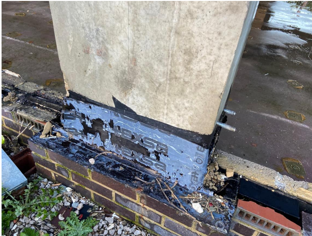
Photograph showing existing membrane and airbrick
