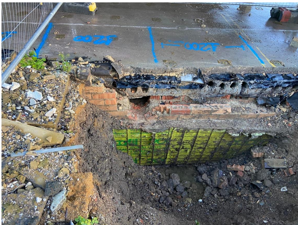
Photograph showing membrane spanning along the outside of the foundation
