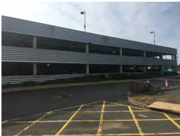
Multi-storey car park in the centre of the Site
