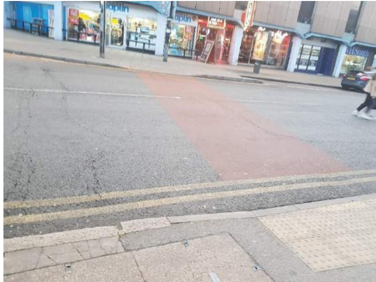
Photo 14 – Informal Crossing Between Belmont Road North and Belmont Road South (L2 and L15)
