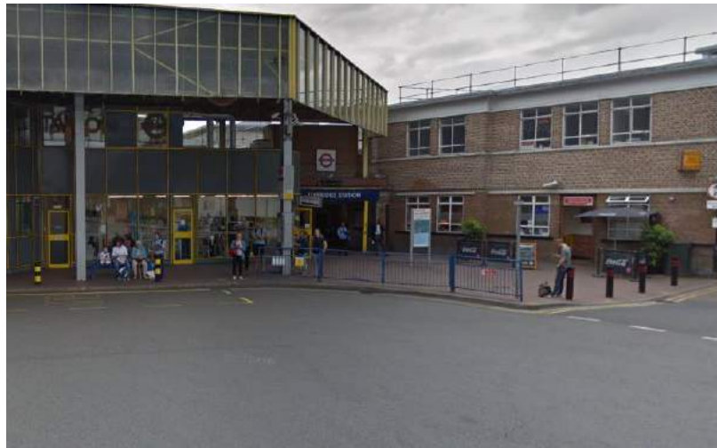
Photo 31 – Exterior of Uxbridge Station
