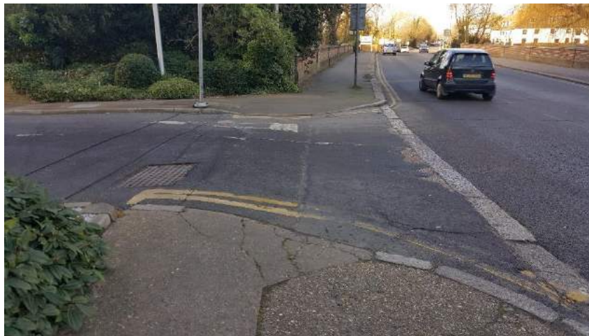
Photo 25 –Junction of Oxford Road/ Site Access (J5)
