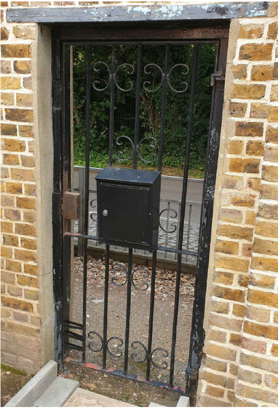
Existing Personnel Gate
