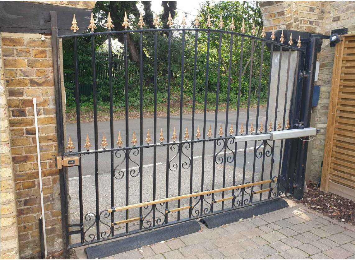
Existing Vehicular Gate
