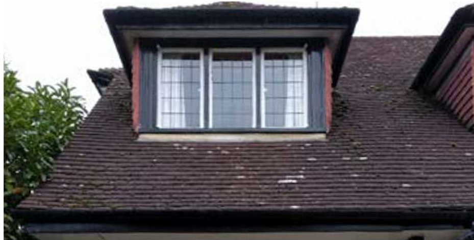
Existing Dormer Window - External
