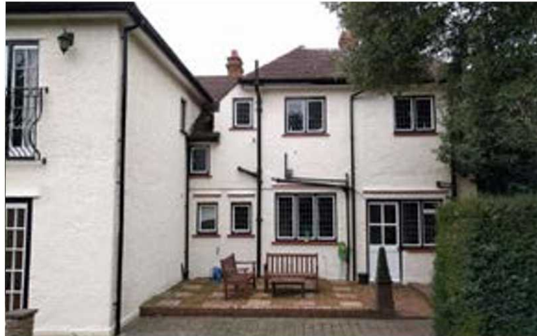
Existing Rear Elevation Window - External
