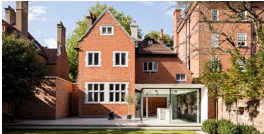
Precedent Image - Finkernagel Ross - Traditional vernacular architecture complemented by a contemporary addition
