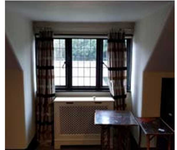
Existing Dormer Window - Internal
