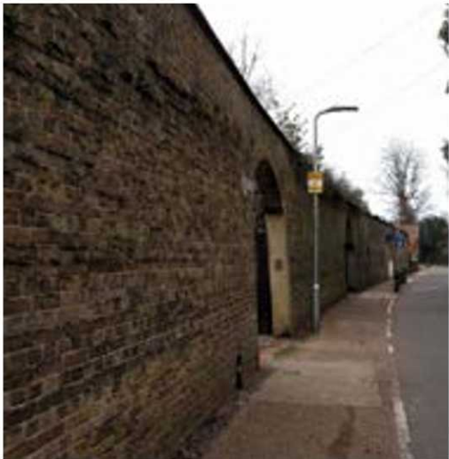
Stretch of the wall between No. 86 and 90 Vine Lane
