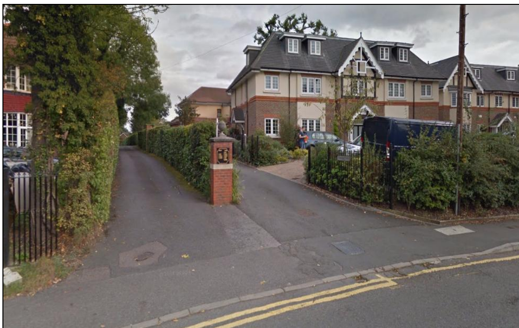
Photograph 2 – Application site viewed from Vine Lane to rear of two large blocks of three-storey apartments
