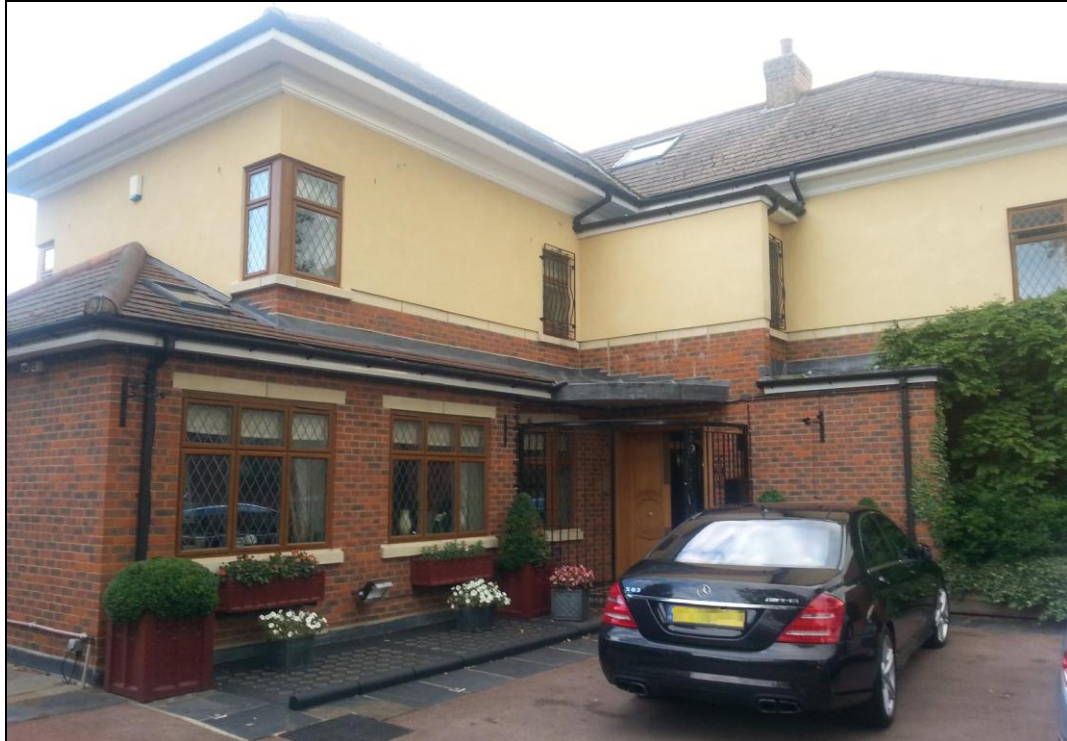
Photograph 1 – Existing house showing location of proposed front extension
