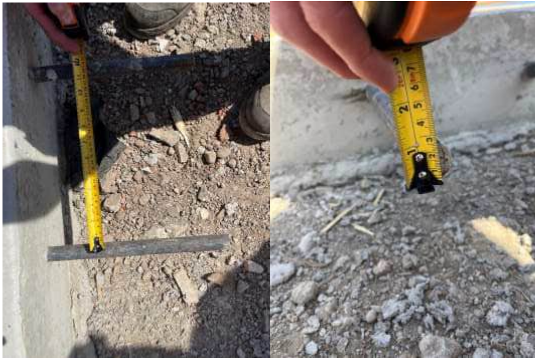
Figure 3 - Dowel Bar Measurements
