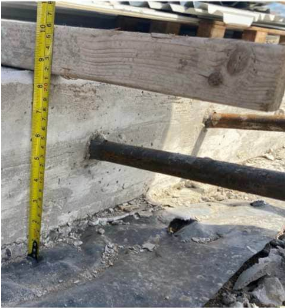
Figure 1 - Concrete thickness measurement
