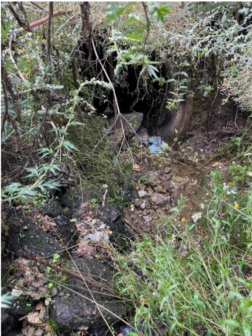
Photo 2. Culvert outfall c.1m diameter
