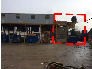
END OF LINE
