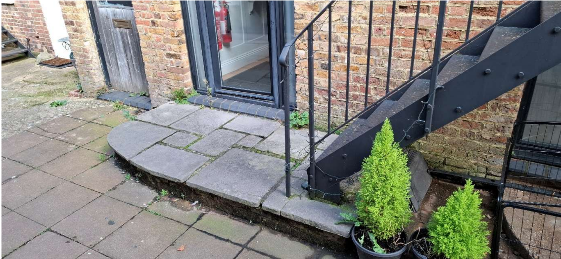
8. RAISED STEP AT PASSAGEWAY ENTRANCE, (STAIRCASE TO BE REMOVED).
