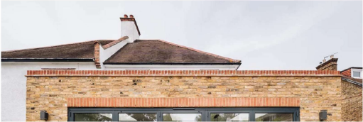
PHOTO SHOWING BRICK-ON-EDGE ON TILE CREASING Rear extension with consealed gutter
