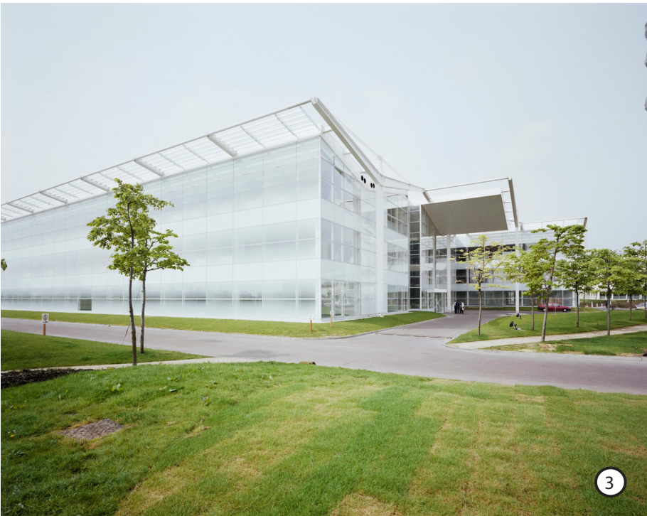
Fig. 6B.6: 1991 Photograph of the Building B3 seen from the north-east along Longwalk Road (Historic England).
