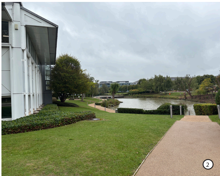
Fig. 6B.5: Pond and landscape seen from Bennetsfield Road looking south. Building A1.1 is to the left.
