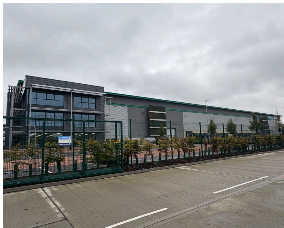
Fig. 4.5: From Iron Bridge Road at the vehicle entrance looking north-east towards unit 1 (DC5). The office block is to the far left.
