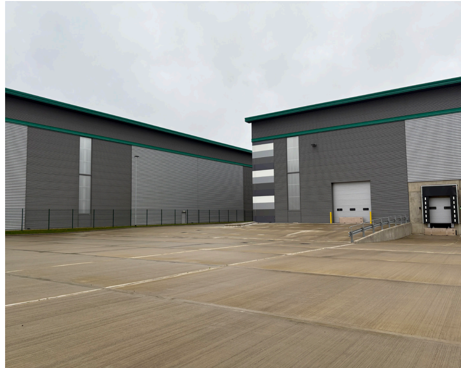
Fig. 4.3: From the north-east yard looking south-west, unit 1 (DC5) is to the left and unit 2 (DC6) to the right.
