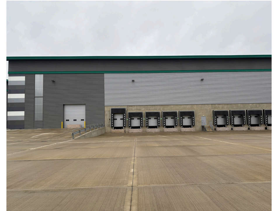
Fig. 4.4: From the north-east yard looking west towards unit 2 (DC6) and loading decks.
