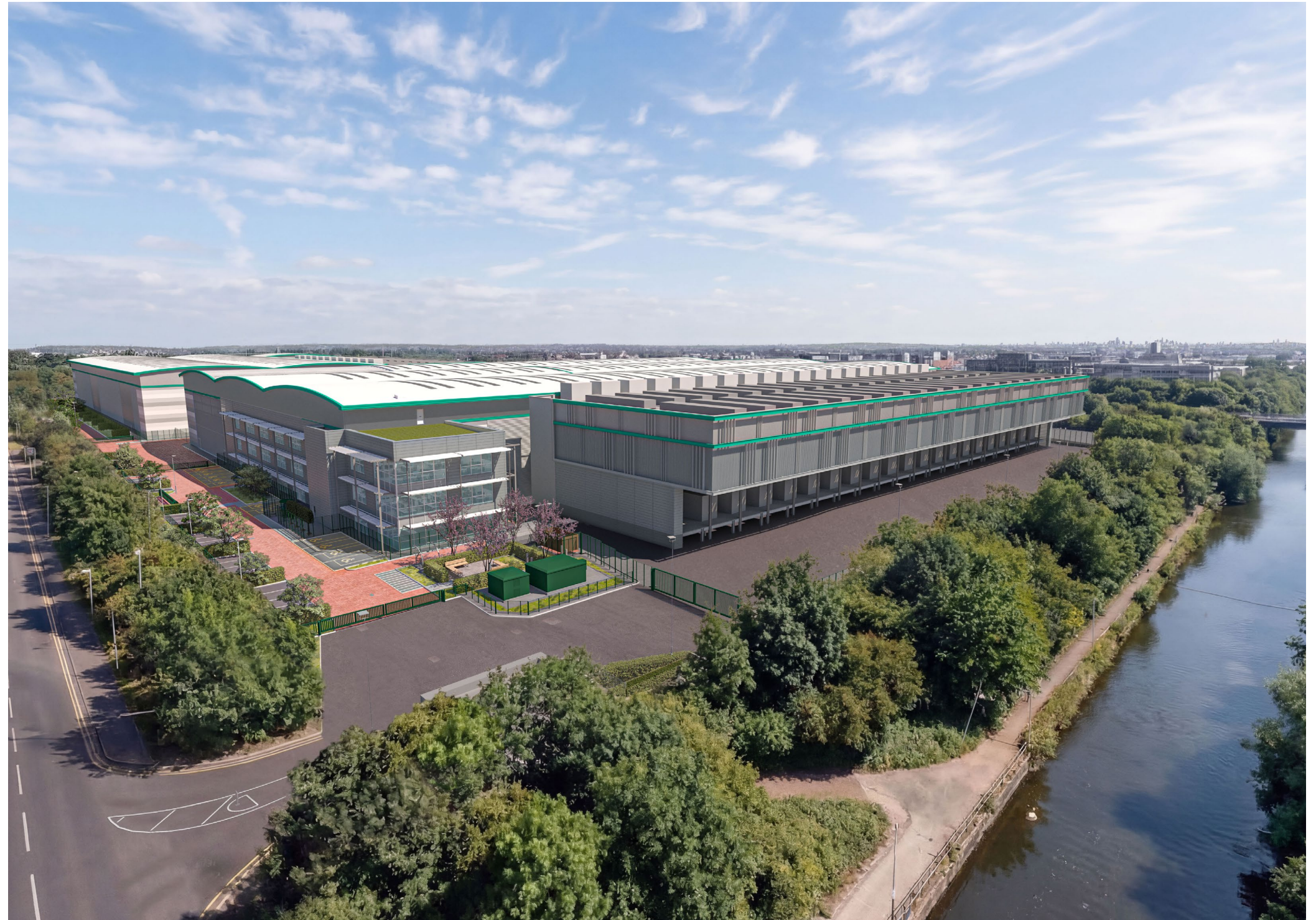
Proposed view from the southwest showing the proposed DC01 gantry in the foreground
