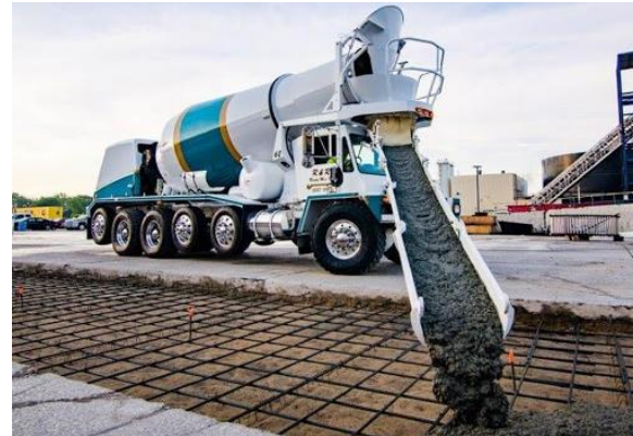
Figure 5.3: An Image of a Concrete mixer truck.
