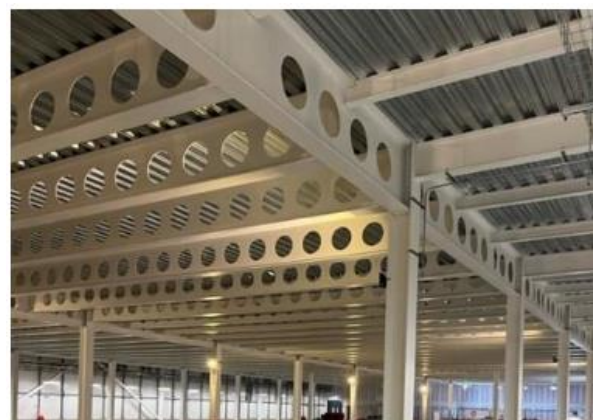
Figure 5.2: An Image of an upper floor structural steel.
