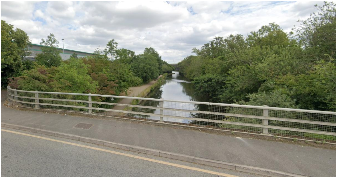
Figure 7 - View of the Grand Union Canal from an Overpass
