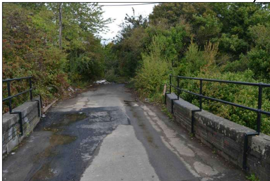
A line of removable bollards to be installed to restrict unauthorised access and fly tipping
