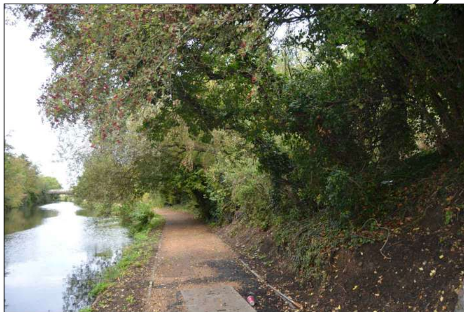
Existing block of vegetation removed and replanted and seeded to improve forward visibility
