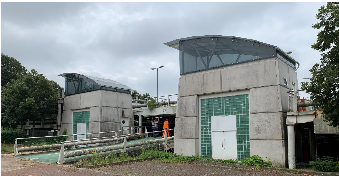
Photograph 3: Multistory Car Park to be demolished
