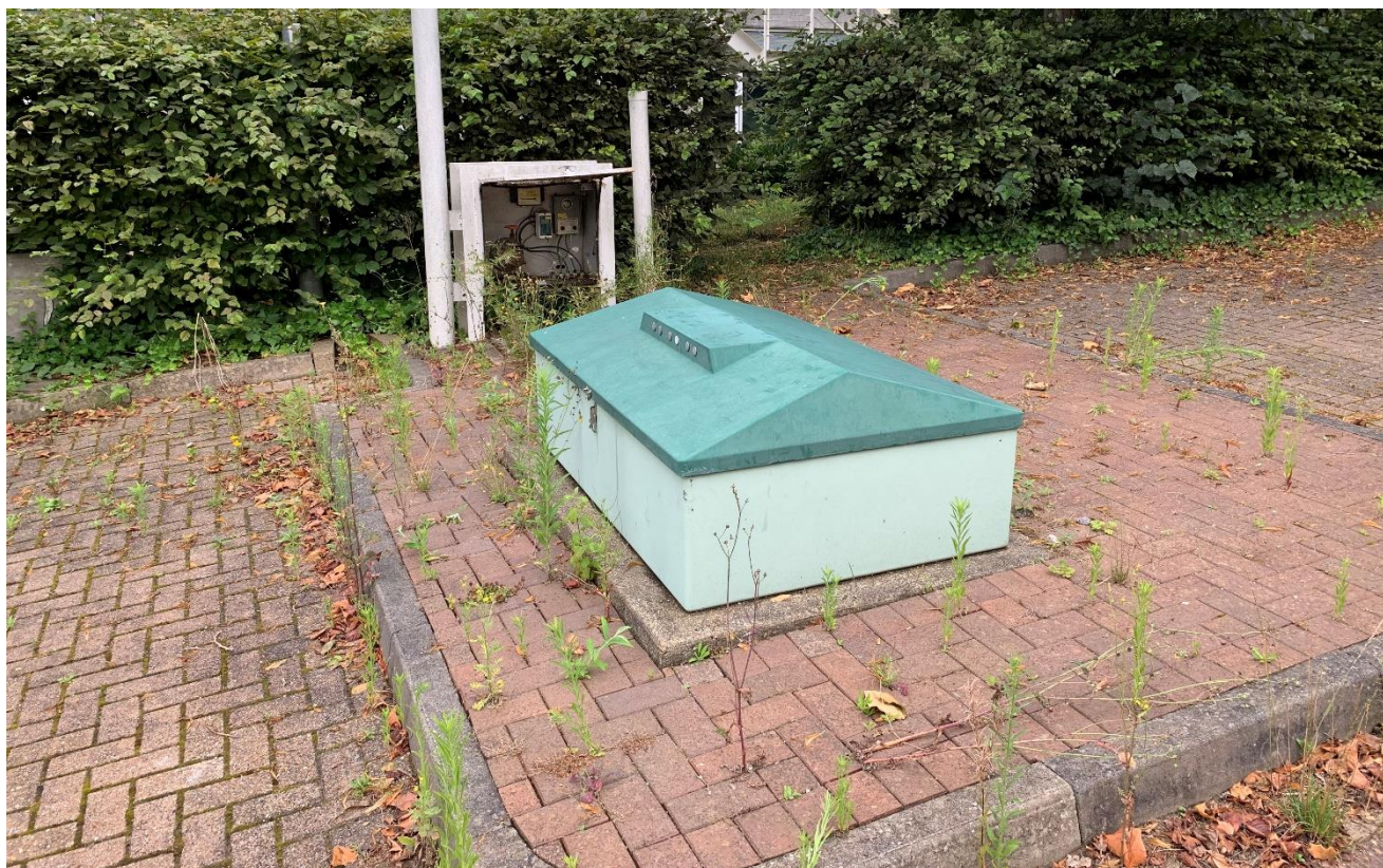
Photograph 4: Below ground tank to be removed
