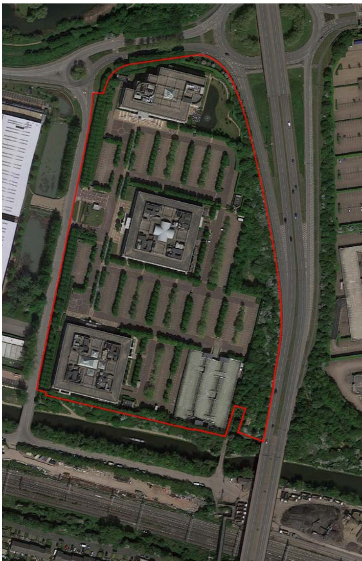
Aerial photo of the application site
