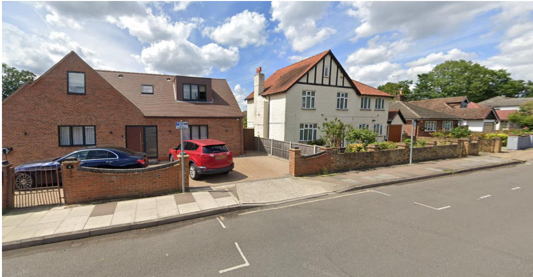
Figure 3: Streetview image of site from Frays Avenue facing north (with No. 16 Frays Avenue visible in the foreground). This view demonstrates how the roof height/massing reduces towards the northern boundary.
