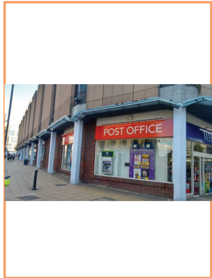
EXTERNAL ATM LOCATION FULL VIEW
