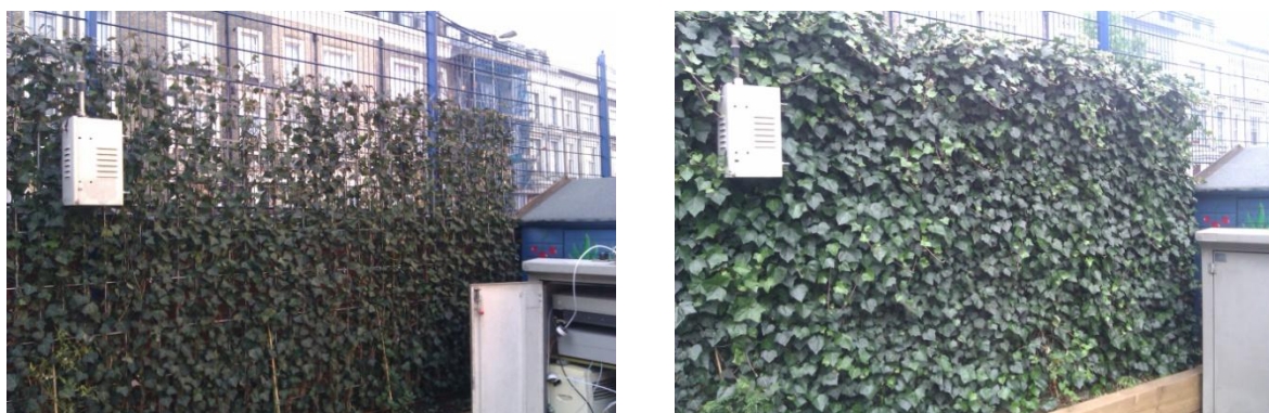
Figure 11: Green screen on installation (left) and after growth period has started (right)
