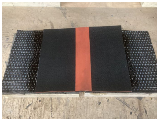
4) Install the Flexjoint over the joint
