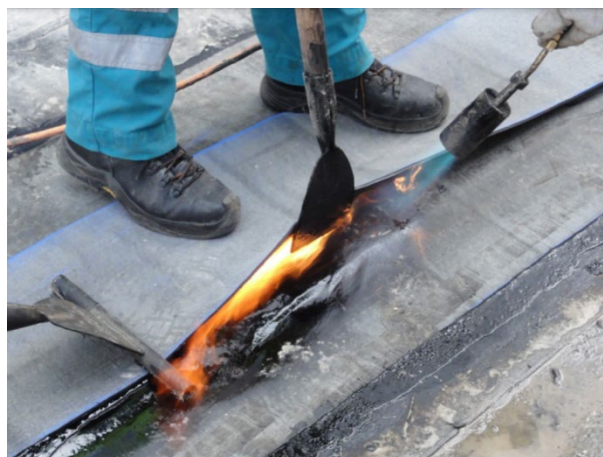
8) The waterproofing cap sheet is torch bonded to the upper side of the joint
