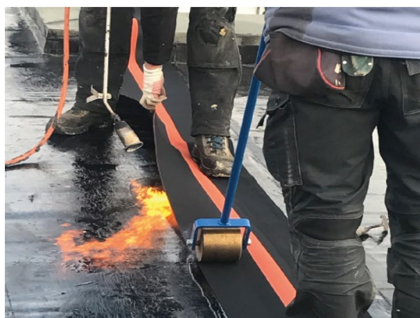
6) Apply pressure using a roller
