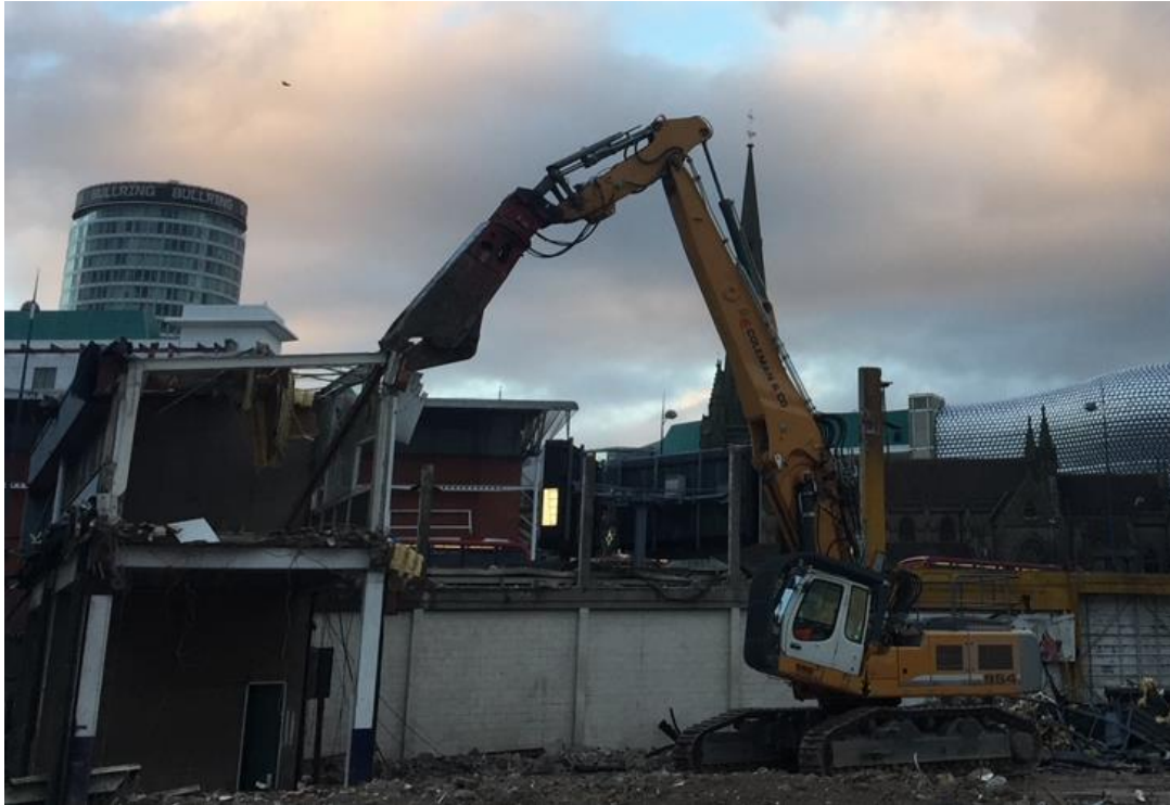
Demolition Excavators with Various Attachments to be Used for Mechanical Demolition
