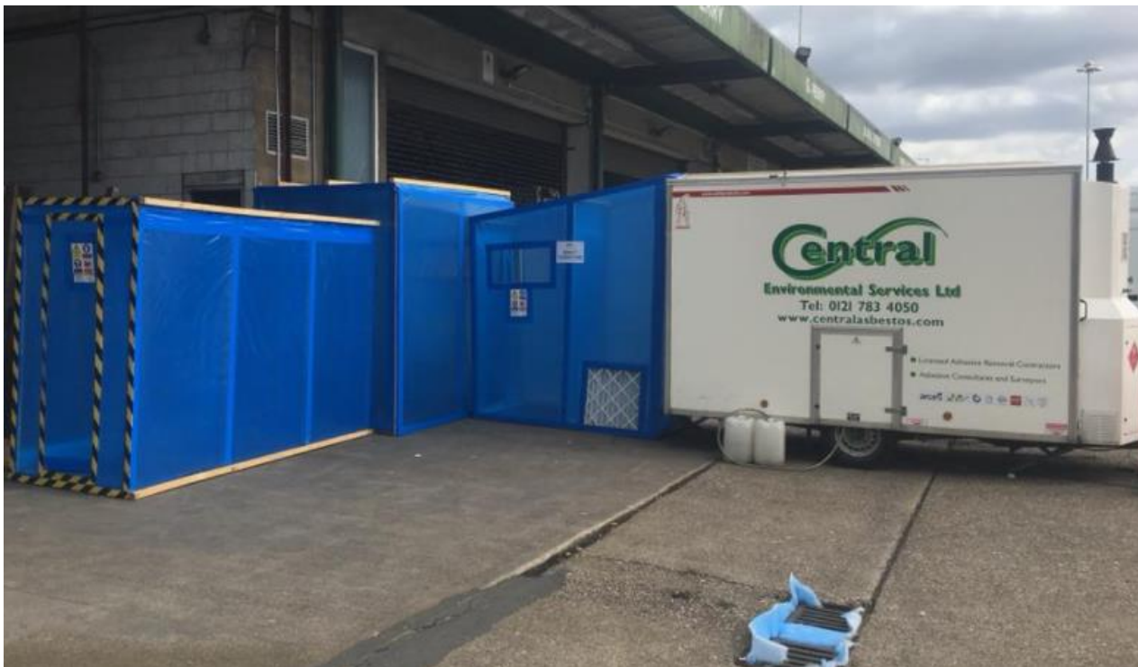
Air Lock to be set up for Licensed Asbestos Removal
