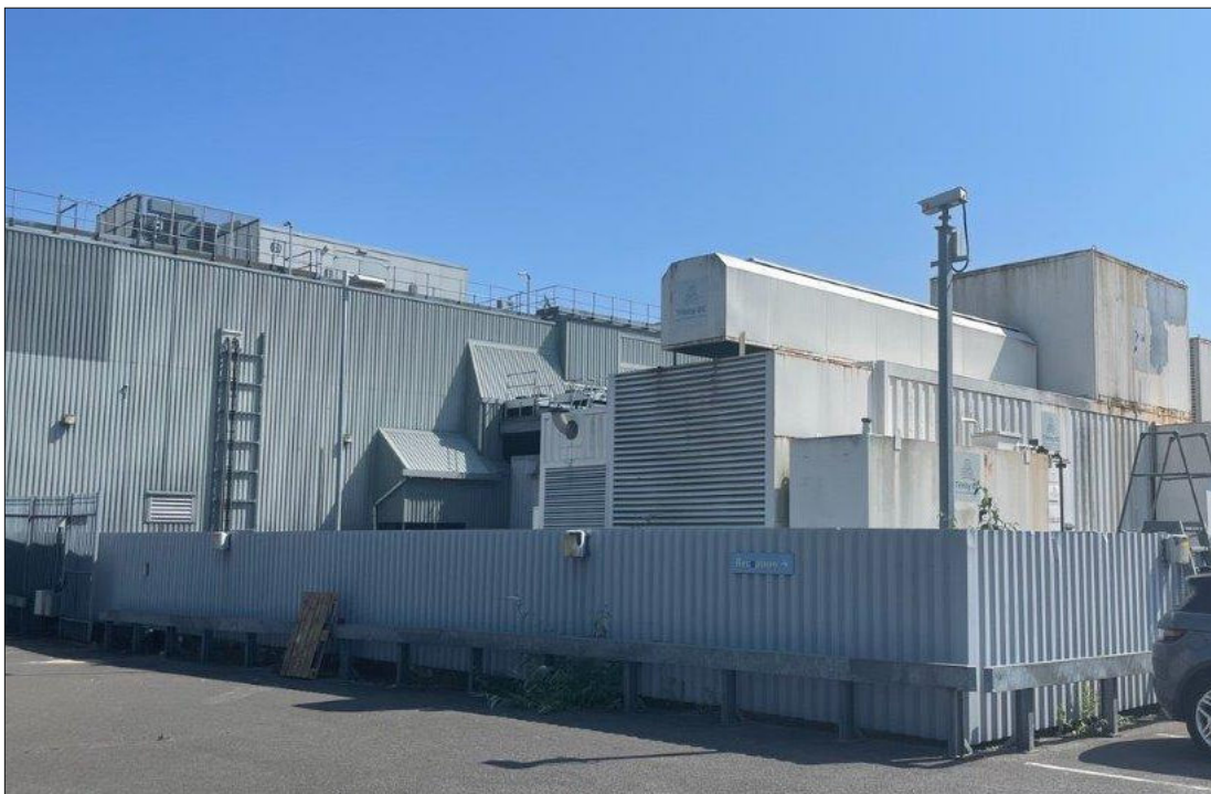
PHOTOGRAPH 2: Exterior of Building B1
