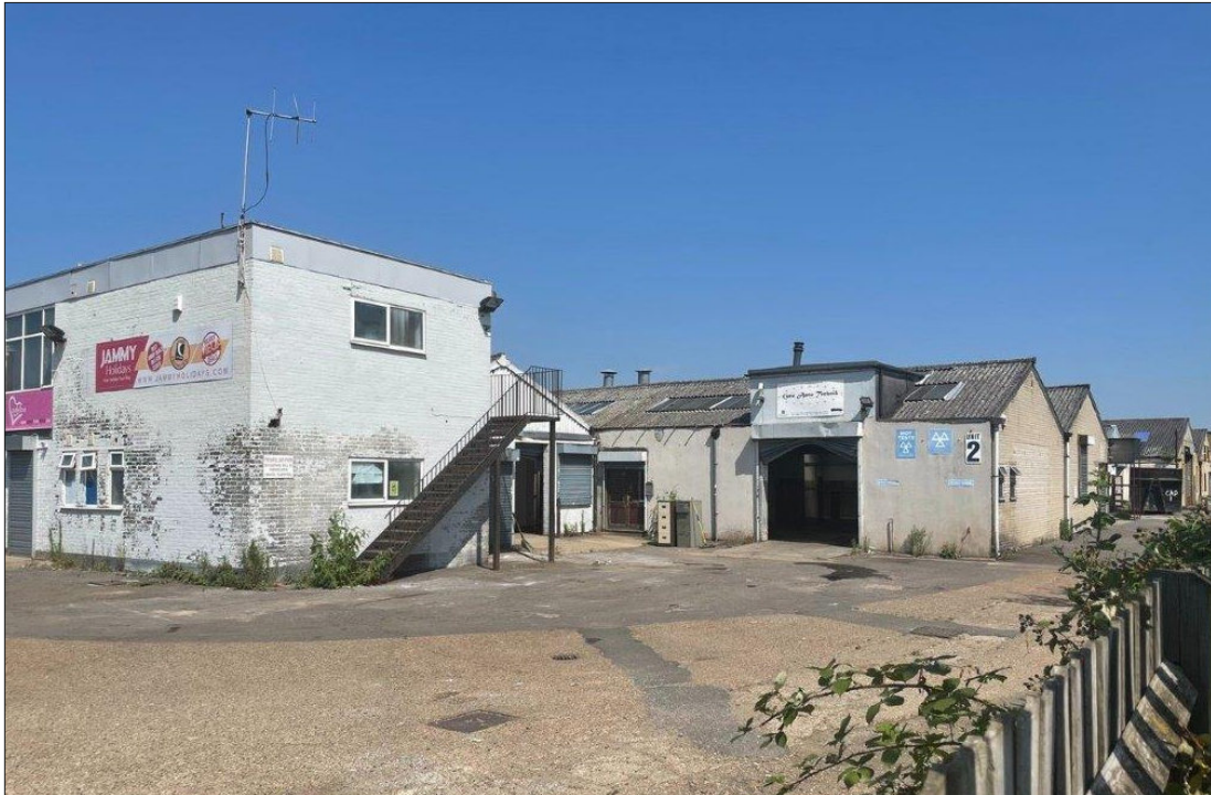
PHOTOGRAPH 3: Exterior of Building B2
