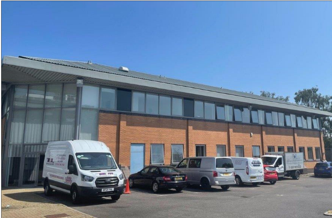
PHOTOGRAPH 1: Exterior of Building B1
