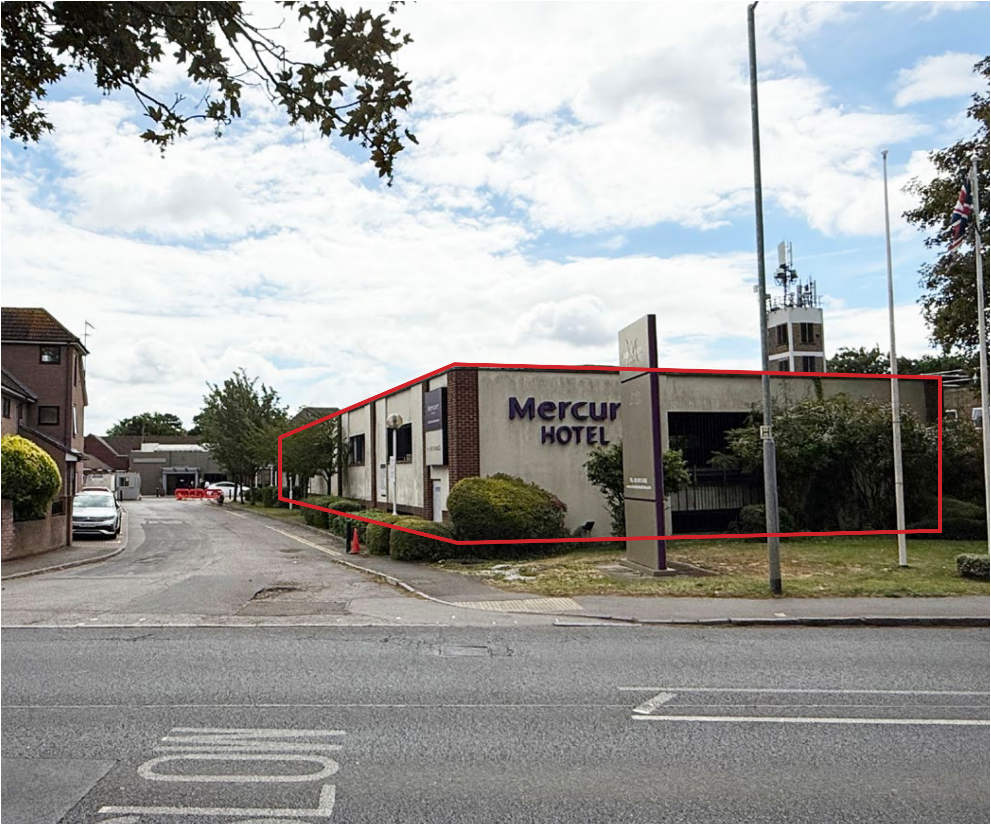
View of the existing building looking east
