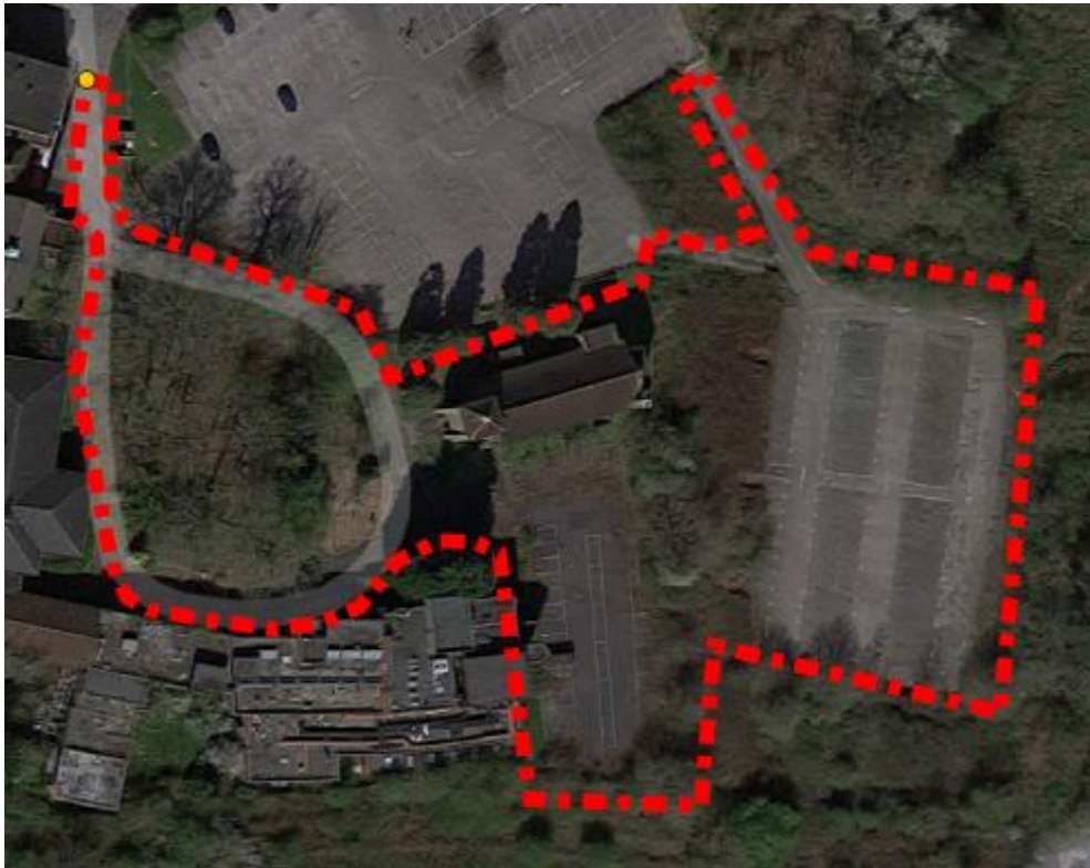
Chapel Car Park (Left) and Access Road and South Overflow Car Park (Right)
