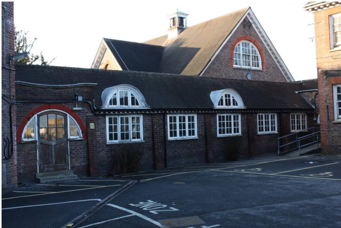
Plate 5: Linking corridor - external view
