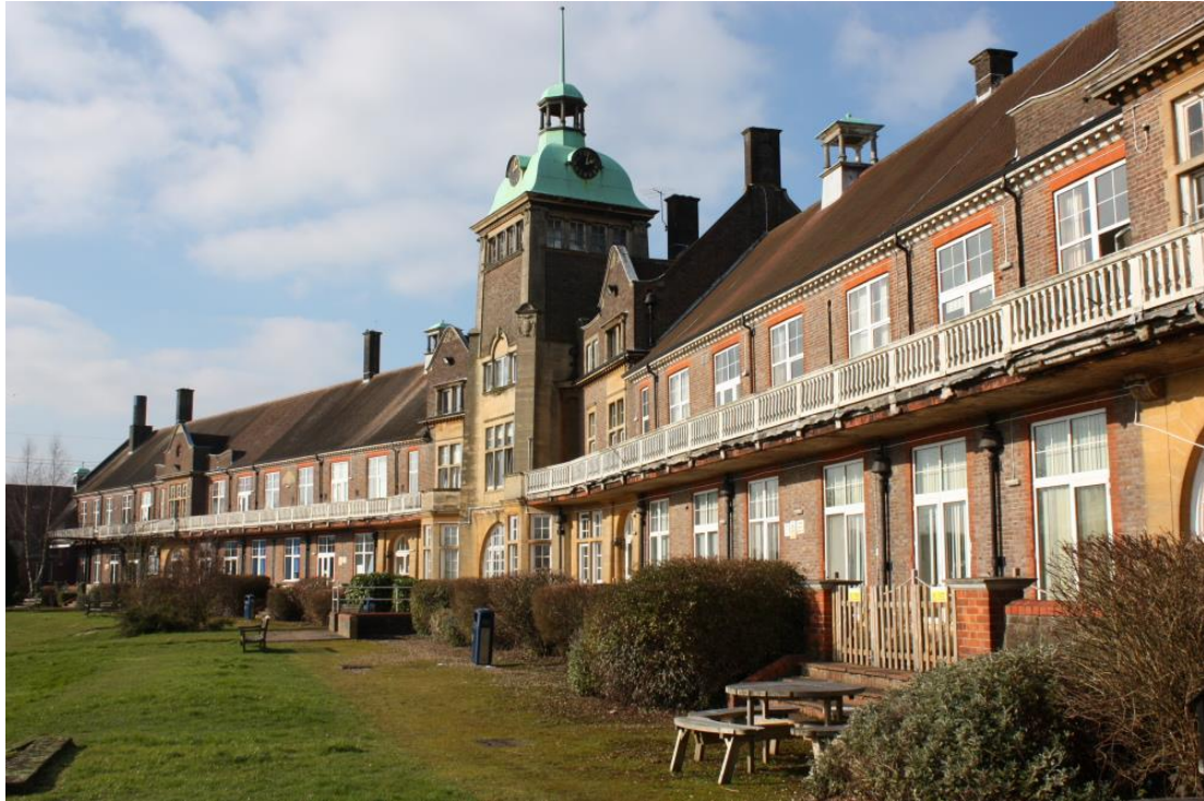
Plate 1: Original V-shaped main hospital ward block (Building 84)
