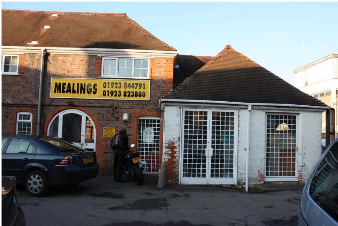
Plate 7: Shop/mini cab base (Building 43)
