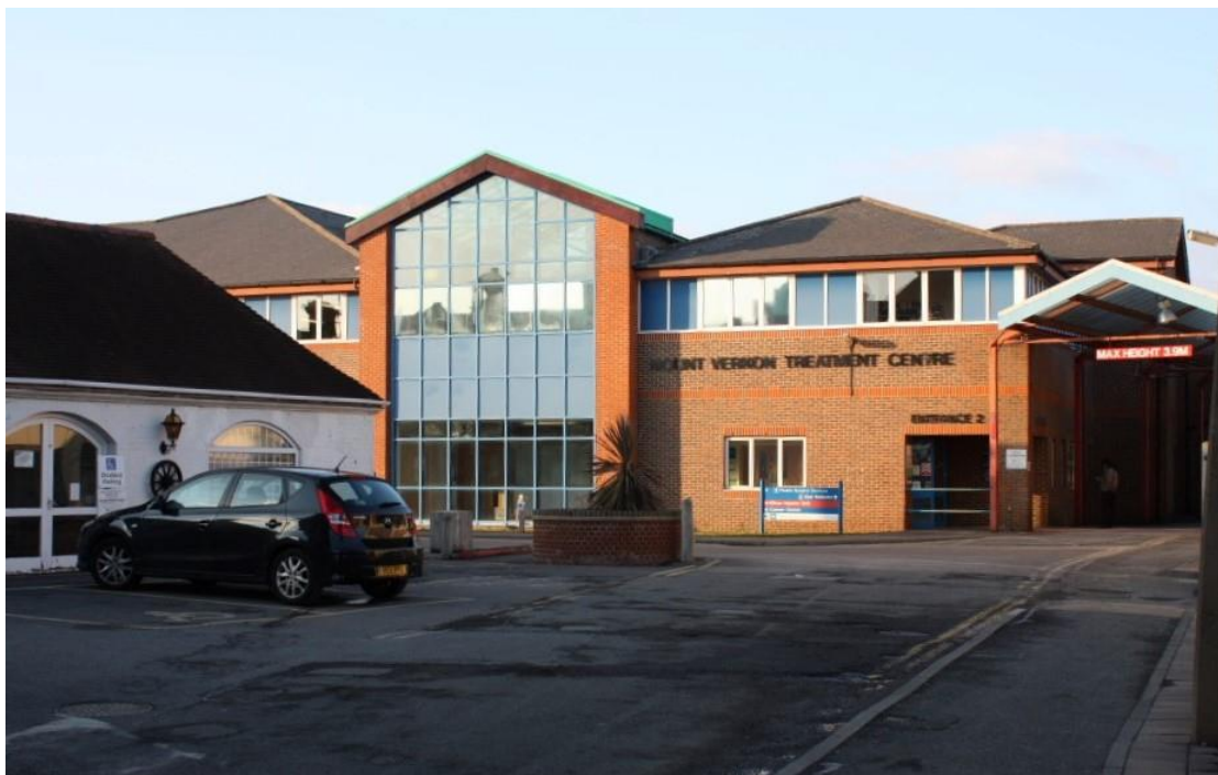
Plate 10: Princess Christian Unit (Building 38) to receive solar panels
