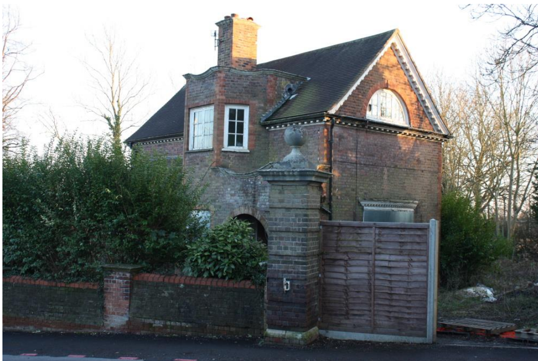
Plate 8: Gate Lodge off Rickmansworth Road (Building 97) and surviving pier
