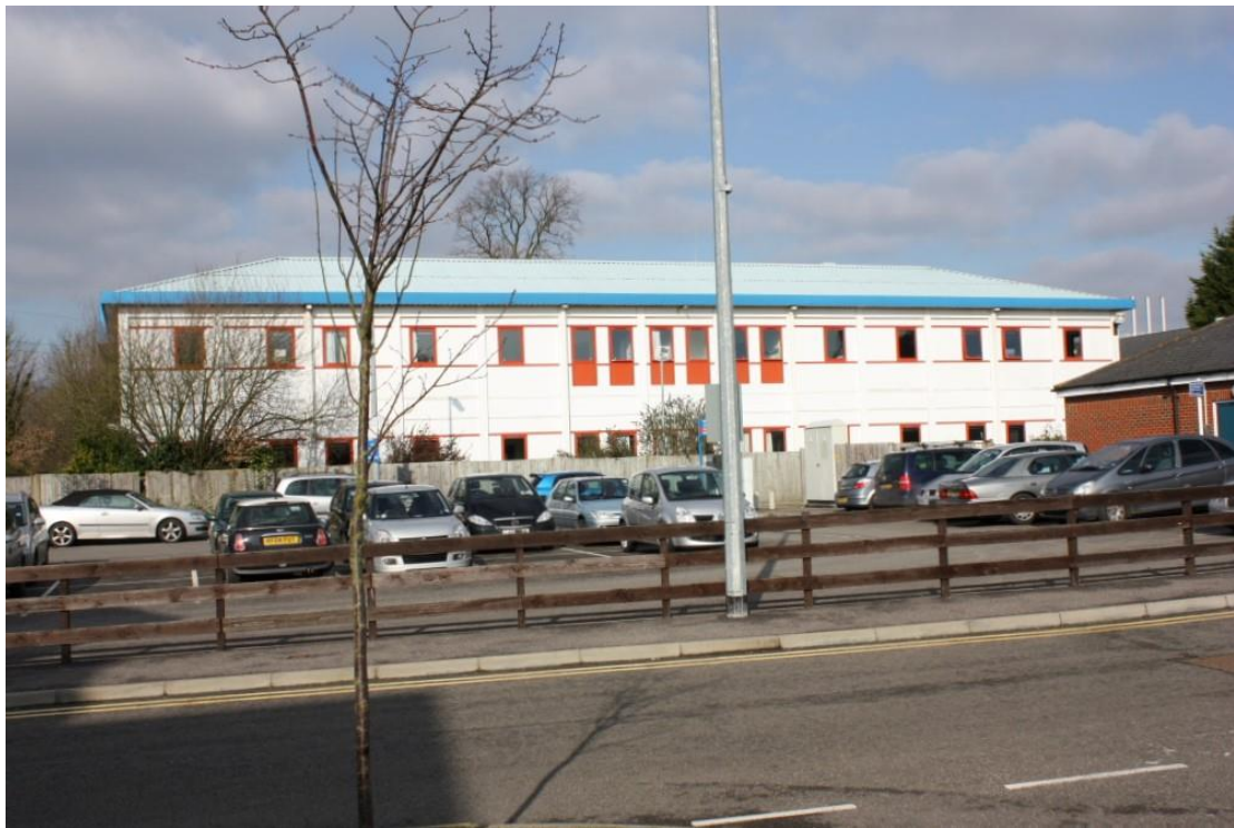
Plate 9: Medical Block (Building 36) to receive solar panels
