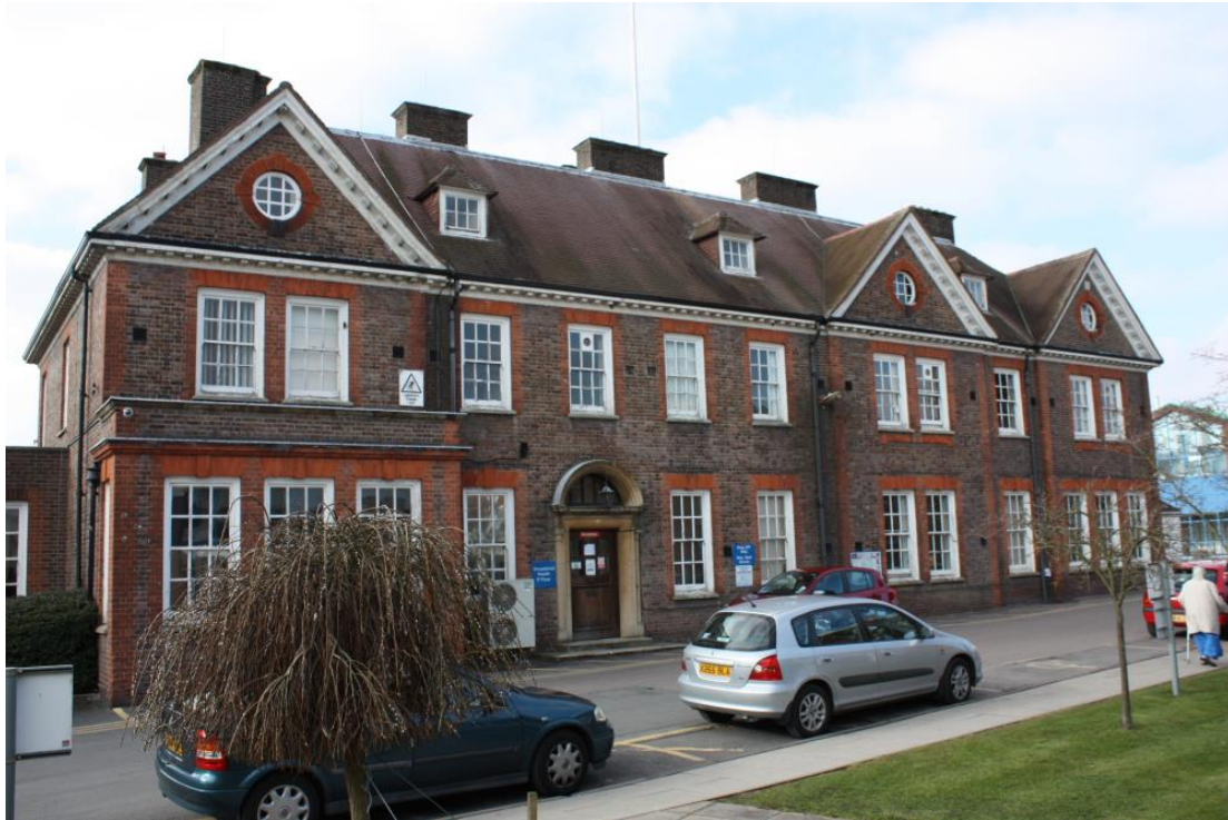
Plate 3: Administration/IT block (Building 54)
