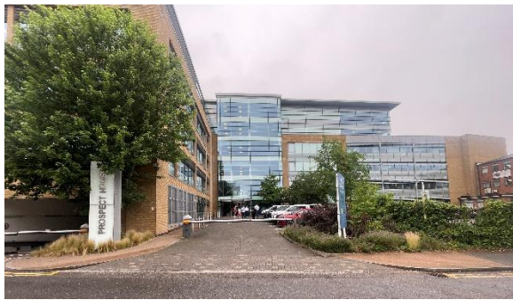
Figure 1. Front Façade and Approach
