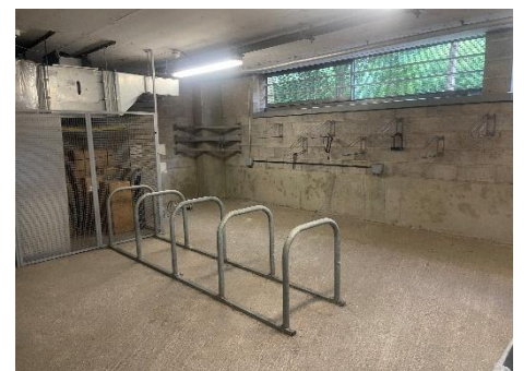
Figure 6. Bike Storage Basement
