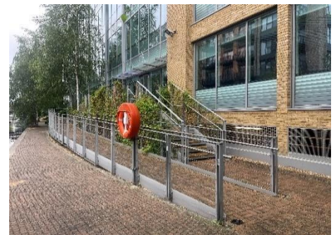
Figure 3. Rear Disabled Access Ramp
