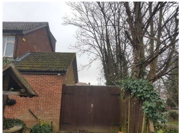
Fig 2: Sycamore immediately adjacent to existing garage
