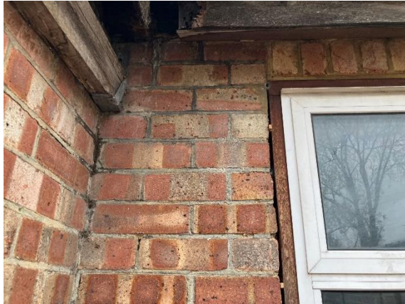
Photo 31: Gap around wooden window frame and rotting soffit/fascia above on 22 St Stephens Road
