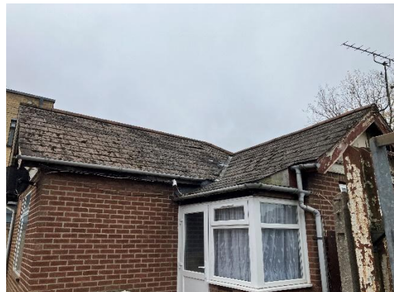
Photo 30: Roof of 22 St Stephens Road with loose and lifting tiles
