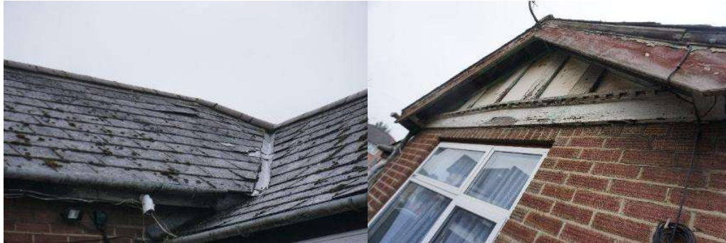
Plate 2: Raised and missing tiles
