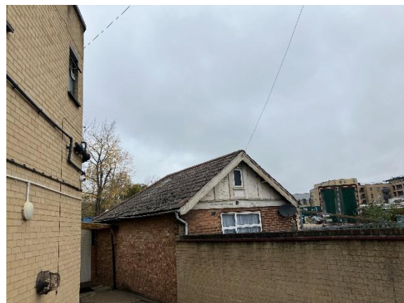
Photo 34: 22 St Stephens Road with missing and loose tiles on the roof
