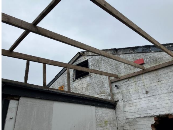
Photo 13: Workshop building and deteriorating roof and absent windows in Unit 6 on Kirby Estate
