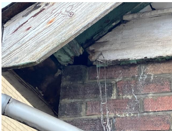
Photo 33: Rotting timbers on the roof of 22 St Stephens Road
