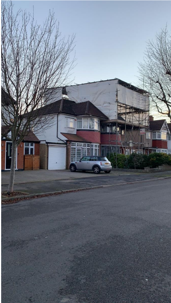
Figure 3: 50 Lowlands Road (Party wall neighbour with 48 lowlands road.)
