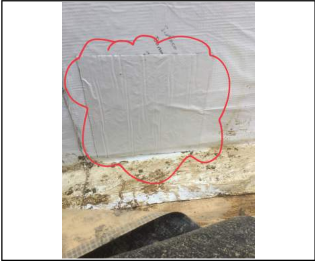
Repair to GRSA Membrane Lift Pit
