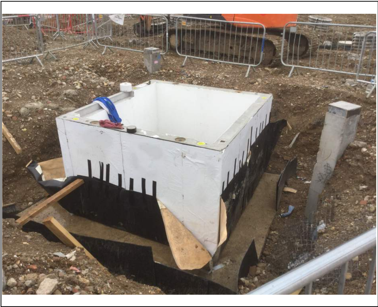
Alternative Overview of Verification Area - Lift Pit 3B
