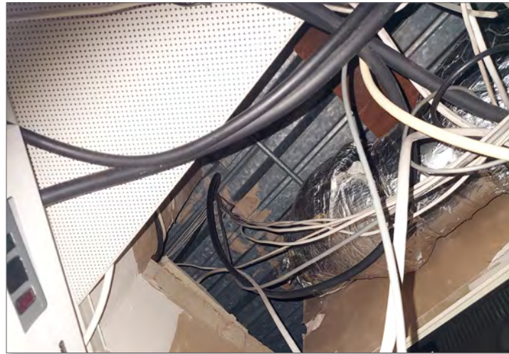
Building 1 Internal view of roof above false ceiling. Showing metal supports and metal roof lining
