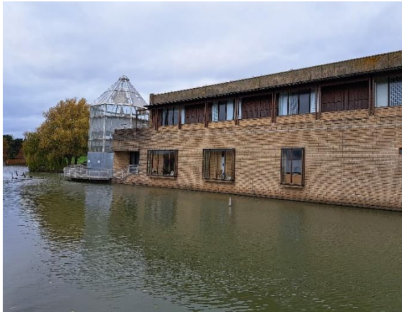
Figure 3.3: The Arena – south elevation and 'Orangery' structure.
