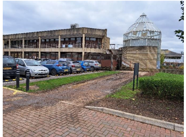
Figure 3.6: The Arena – north elevation with staircase, bin store and 'Orangery'.
