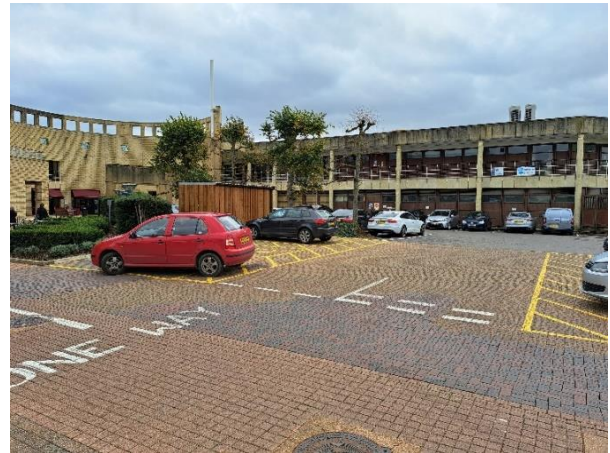
Figure 3.4: The Arena – north elevation and Rotunda.
