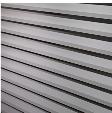
Powder coated Plant Louvres set within the existing Wall.
