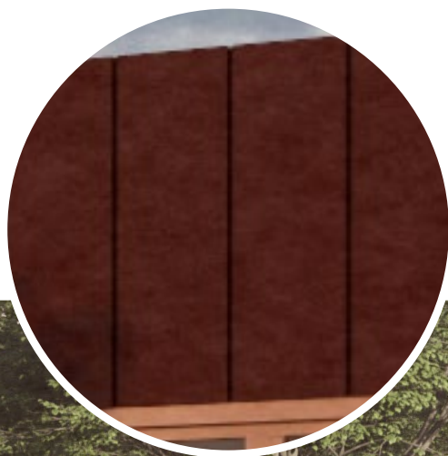
COMPOSITE METAL CLADDING
