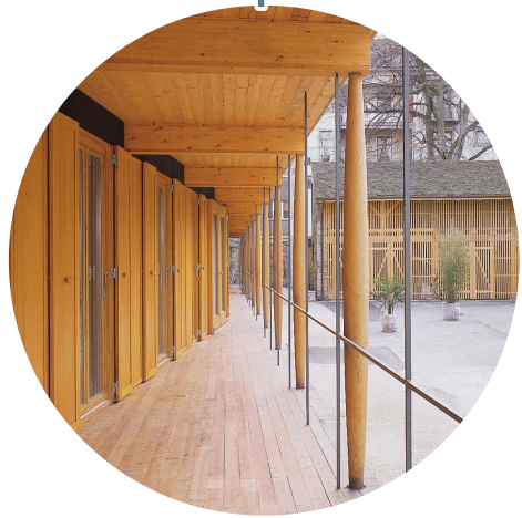
LIGHTWEIGHT TIMBER SPINDLE SUPPORTS
