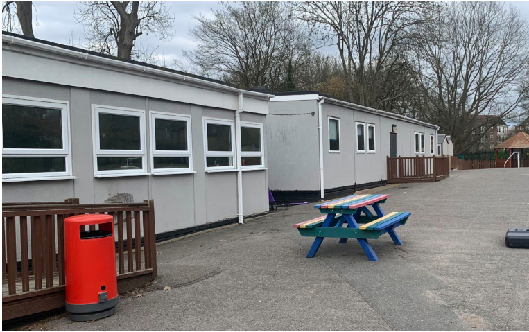
Porta cabins removed in 2021
